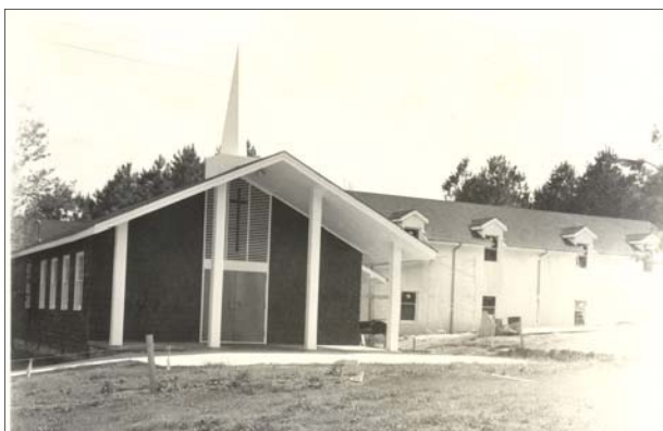
St. David's in 1975 when the "new education wing" was being built.
